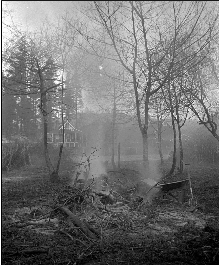
Burning brush with Girling home visible in background, between 1912 and 1928 (2008-025-641)
